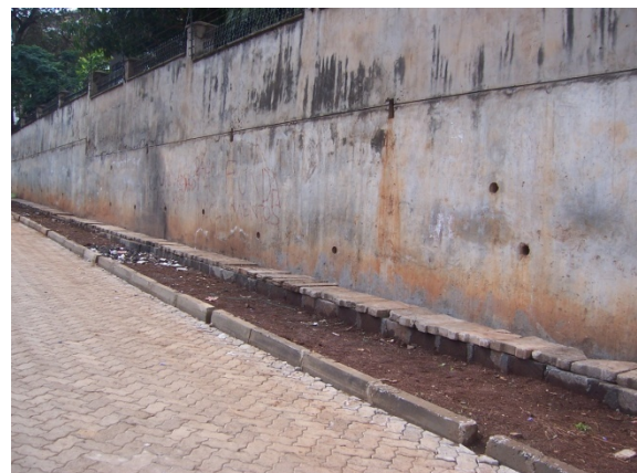
Plate 1B: Road reserve (formerly as shown in Plate 1A as farm) converted to road (Parita Shah 2017)
