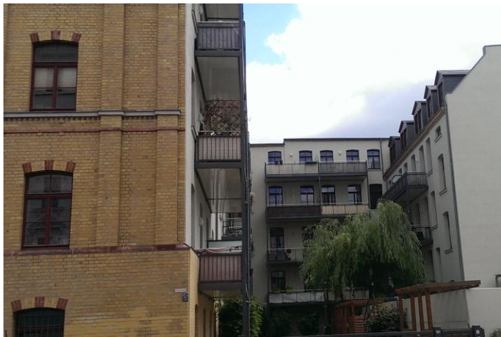
Fig. 17: Example of balconies attached at the Lene-Voigt park quarter own photograph
