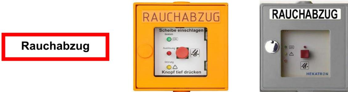
Sign marking a button for the smoke extractor (sample)
